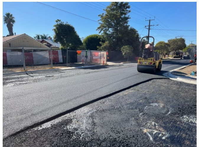
New asphalt pavement at the Harvey Avenue crossing
