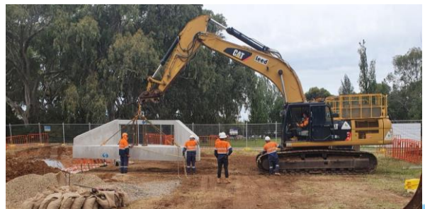
Above: Positioning the headwall
