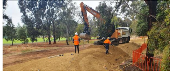
Above: Trimming the edges of the containment mound
