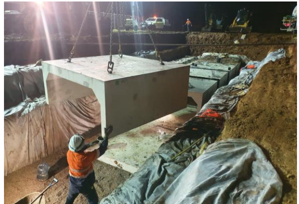
Above: Lifting in the culvert crown
