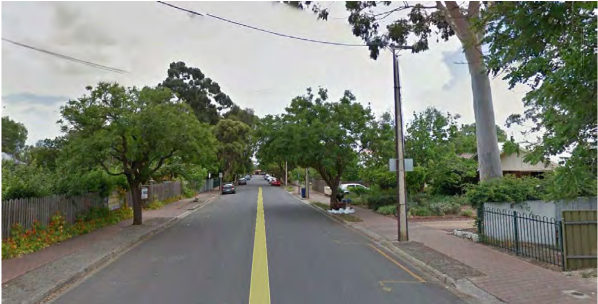
Photo 2: View of the Fern Avenue Culvert Crossing
