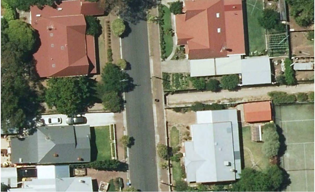
Photo 4: Aerial View of the Torrens Avenue Culvert Crossing Location
