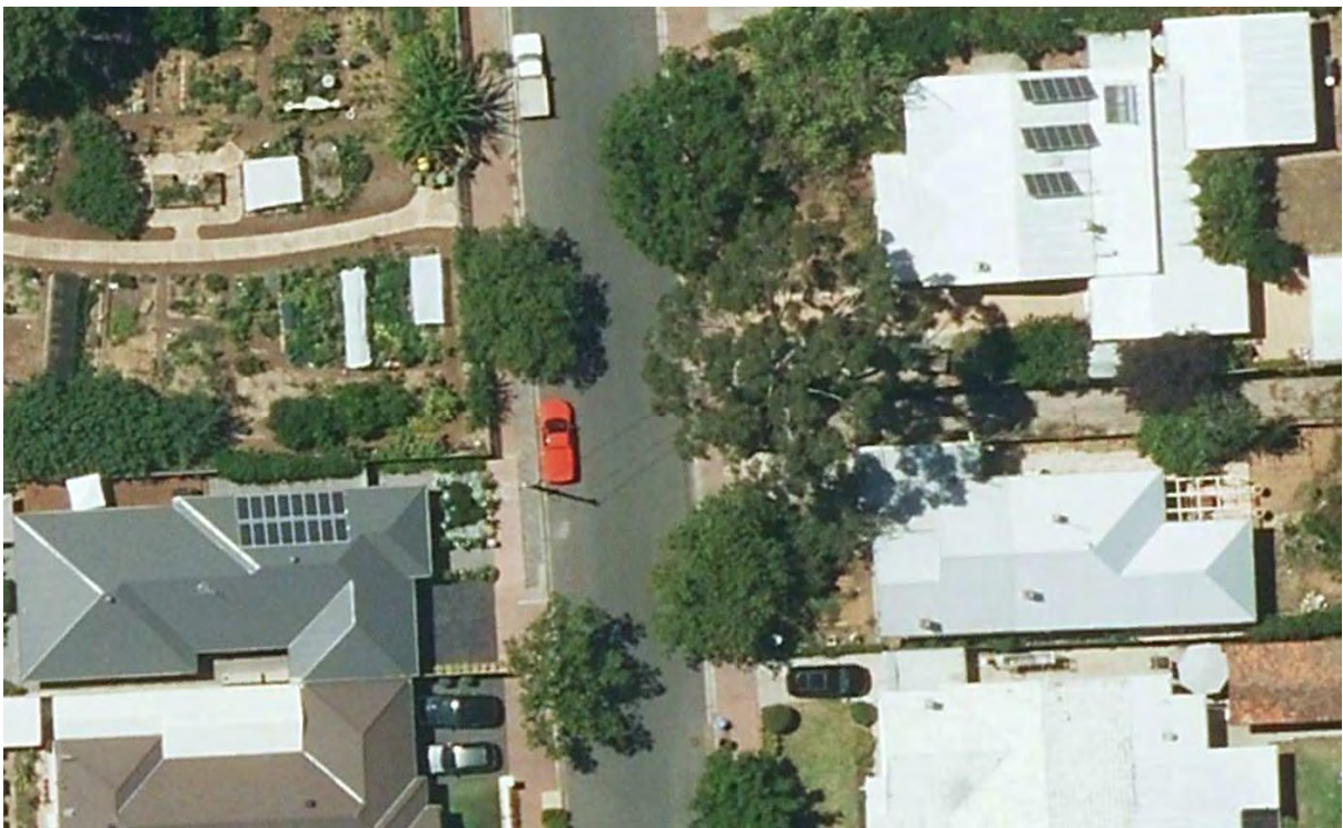
Photo 3: Aerial View of the Fern Avenue Culvert Crossing Location
