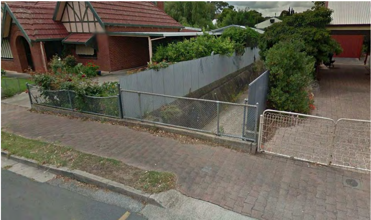
Photo 1: View of Eastern Side of the Torrens Avenue Culvert
