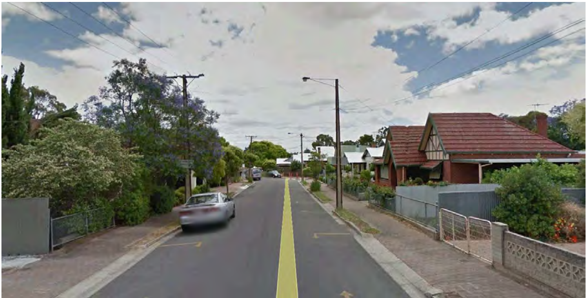
Photo 3: View of Torrens Ave Culvert Crossing
